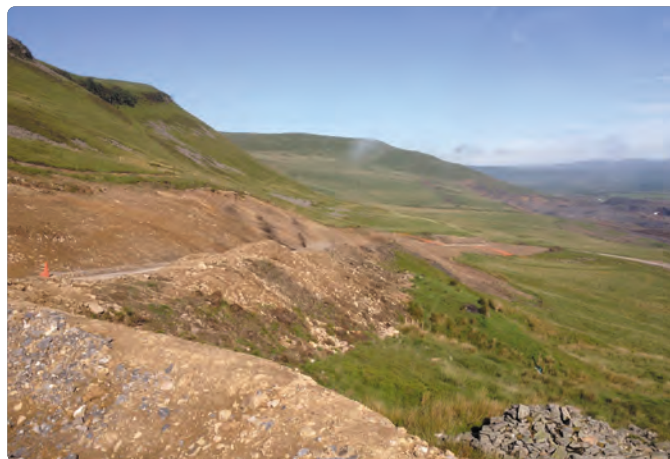
Pennant Walters: Works associated with the HMP at Mynydd Bwlfa Wind Farm
